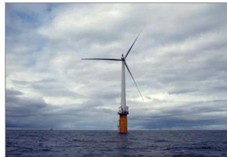
Hywind I Floating Turbine (Statoil, Norway)
