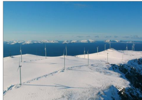
Havøygvælen Wind Farm (Artic Wind, Norway)
