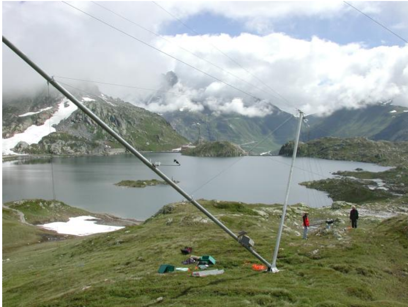
Installation of a met mast in the alps
